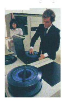
First Disk: IBM 305 RAMAC (1956) 5MB capacity 50 disks, each 24"
